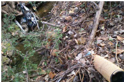
SEWER MATERIAL AND TRASH IN CREEK
