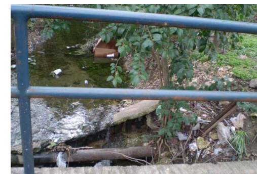
TRASH (LOOKING SOUTH FROM E AVE I BRIDGE)
